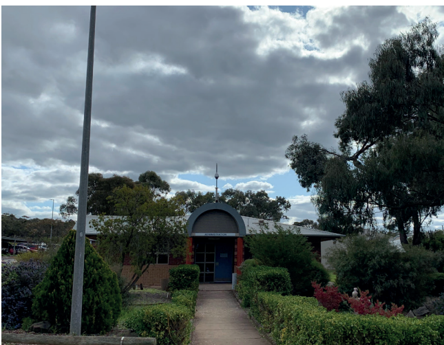
The facility incorporates a mix of prison cells as well as independent living units.
