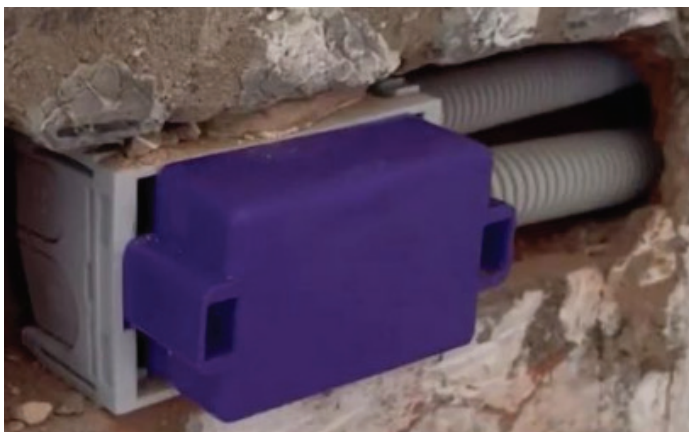
Safe install ready for plastering.
