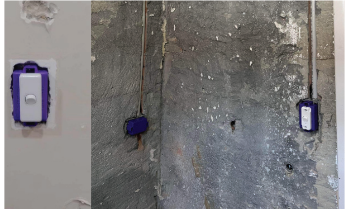
Safe temporary switch lighting.
