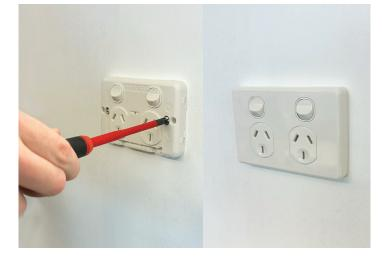
Level the grid plate and tighten both fixing screws with a standard Phillips head screwdriver. Attach the cover plate
