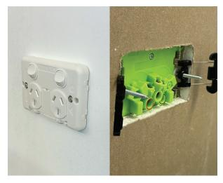
Insert the grid plate into the aperture, releasing the clamps at the same time. The clamps should adhere to the back of the plasterboard.
