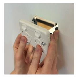
Remove the cover plate. With both hands hold the grid plate while pressing both the spring-loaded clamps approx. 30mm inwards. Do not bend any further.
